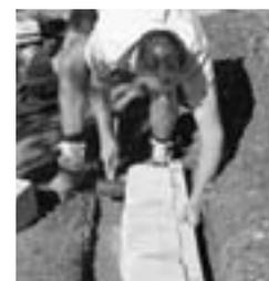
Handy Tips: Use a rubber mallet to tamp blocks into place - a metal hammer may crack them.
